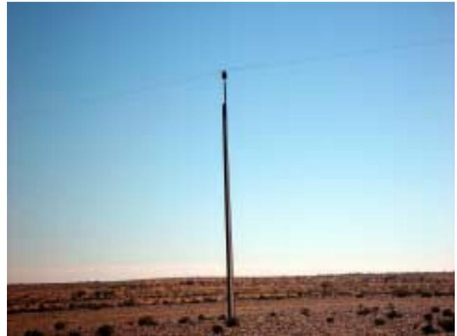
**Photograph No. 2 – Single Conductor 19 kV Circuit with Earth Return**
