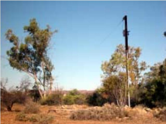
**Photograph No. 1 – Single Phase Service in South Australia with Earth Return**
