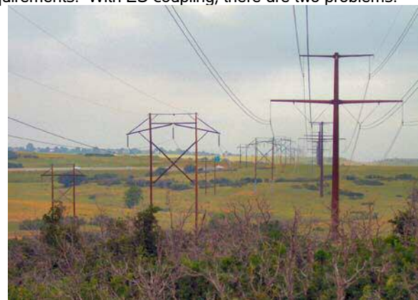
Fig. 7. Three Lines Sharing One Right-of-Way
