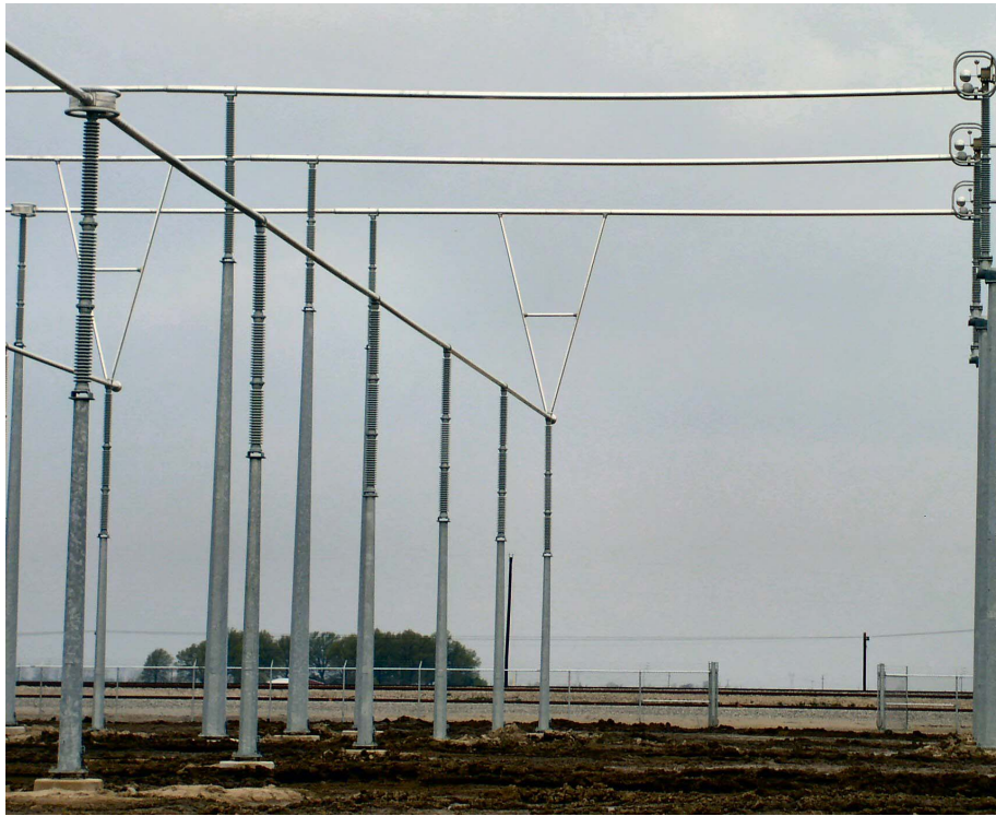
Figure 2: Deflection in 60 ft. bus span.
